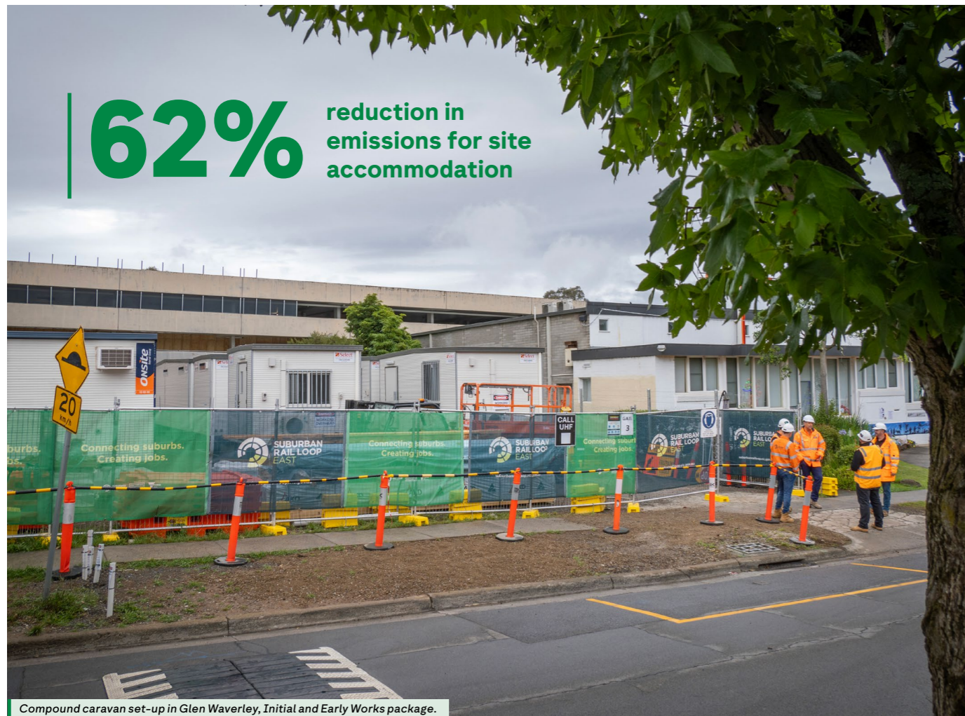
Compound caravan set-up in Glen Waverley, Initial and Early Works package.
