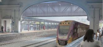
The trusses (large metal beams that support bridges) reference the historic trusses in the train hall roof. Known as Pratt trusses, they combine vertical and diagonal geometry.
