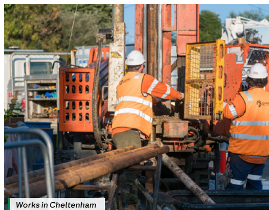
Works in Cheltenham
