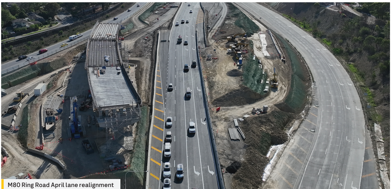
The retaining wall under construction along Service Road in Watsonia
