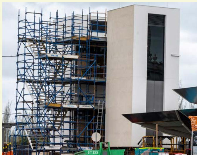
Lift fit-out works underway on the ground before the 'Big Lift'.
