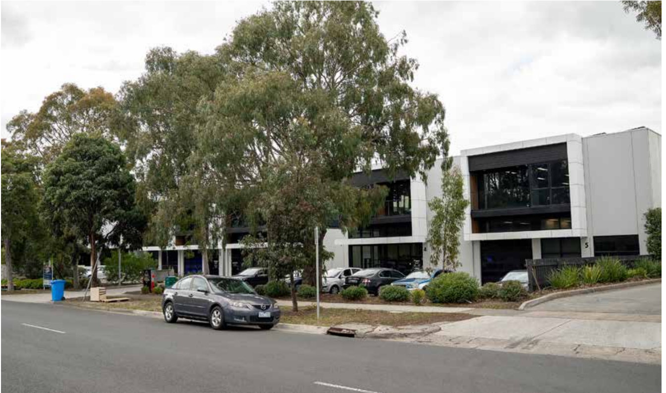
Existing industrial buildings in Bayside Business District
