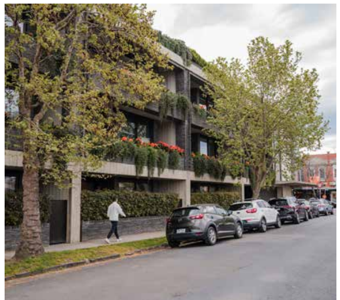
Apartment building, Pine Avenue, Elwood
