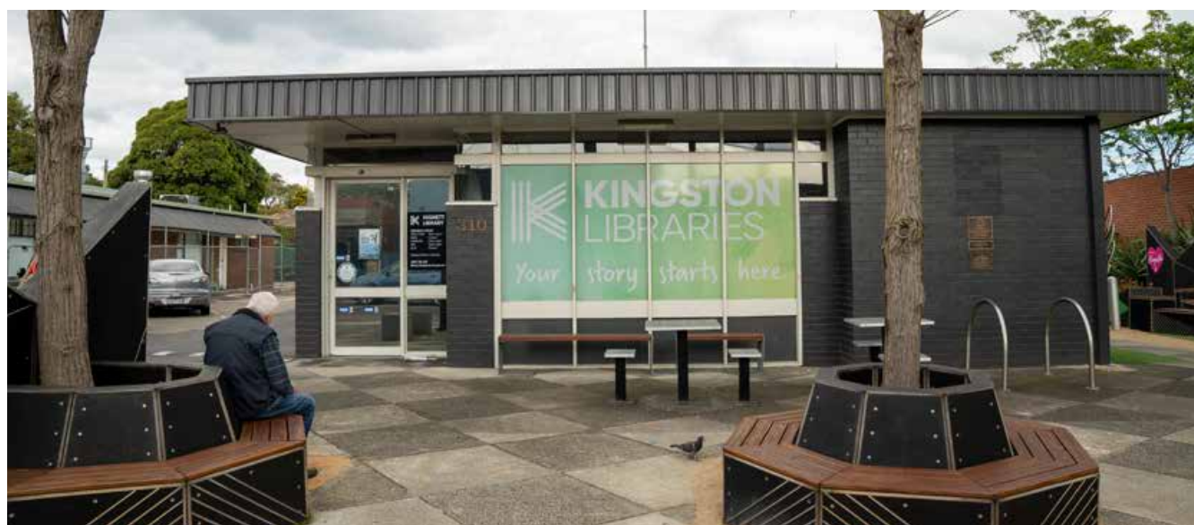
Existing Highett Library and its forecourt
