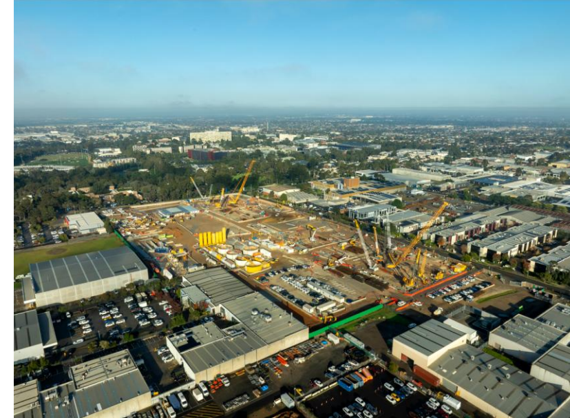
Monash SRL station site: Diaphragm wall construction underway
