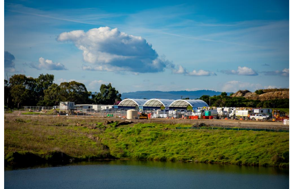
Site sheds and offices
