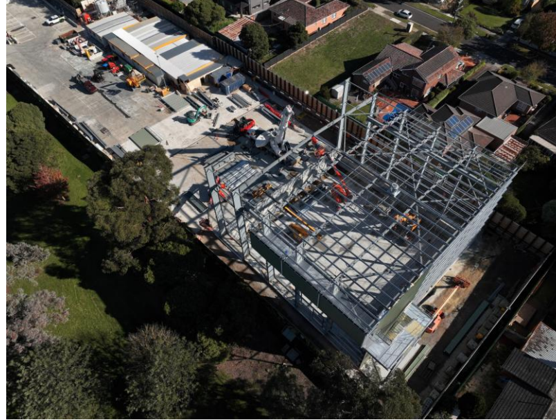
Mount Waverley emergency support facility: acoustic shed under construction
