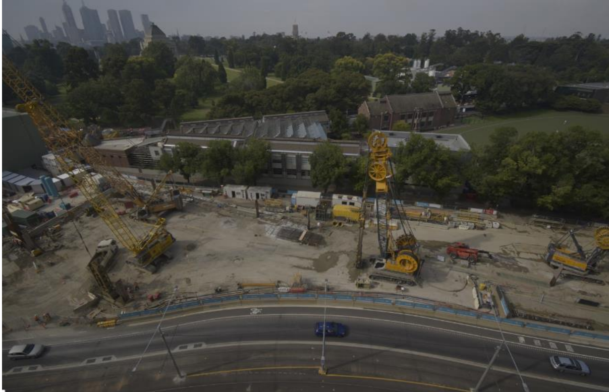
D-wall and piling works underway in middle box
