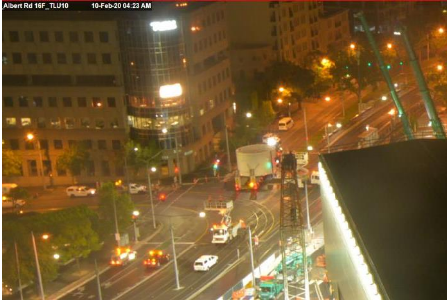
TBM Tailskin Delivery 10/02 – 4:00am
