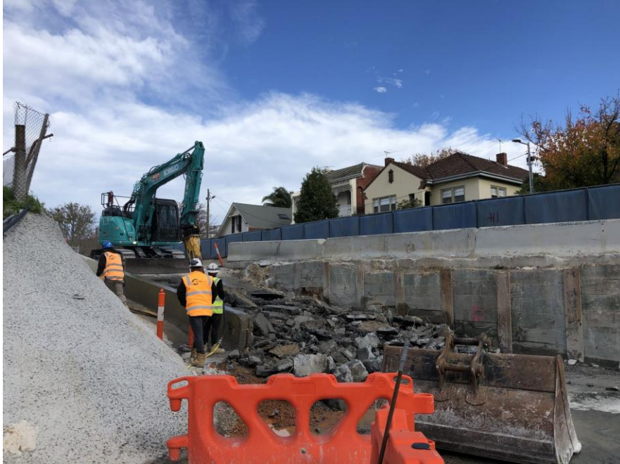
Ramp modification works in May
