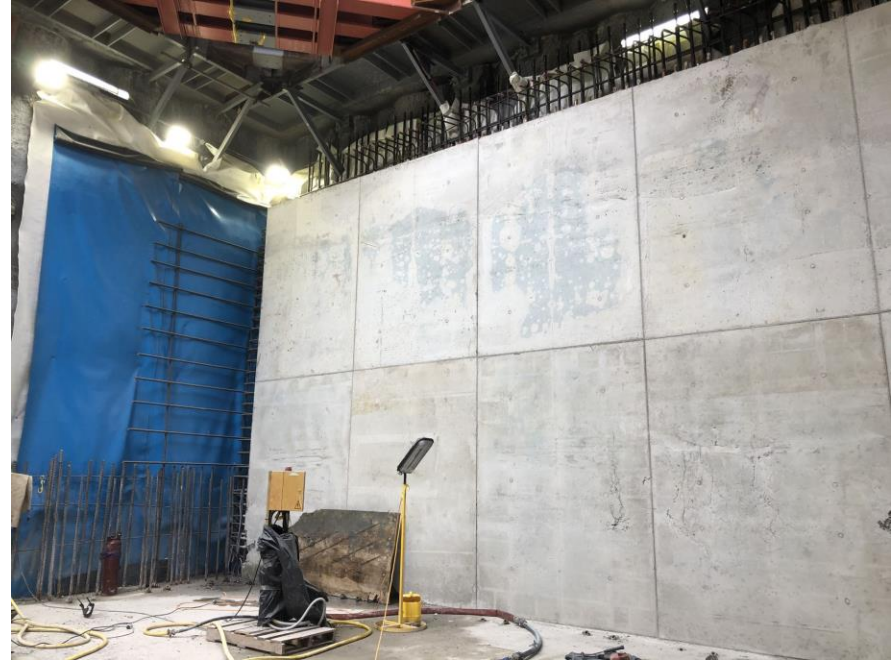
Completed structural wall on northern end of the retrieval shaft
