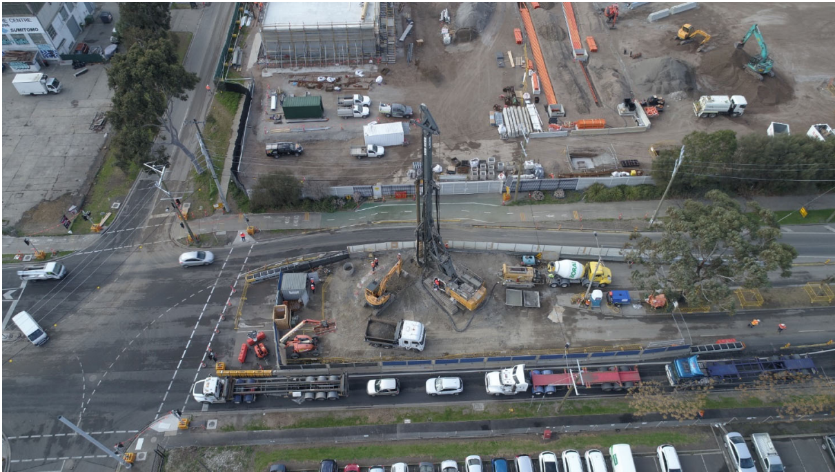
Photo 1 – Piling works on Whitehall Street – North (Source: WGTA)
