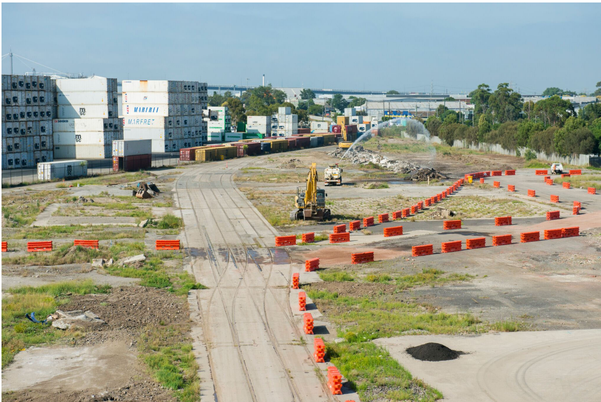
Photo 4 – Spoil management and site delineation – North (Source: WGTA)
