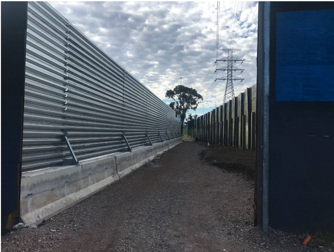
Photo 2 – Temporary noise walls – West (Source: WGTA)
