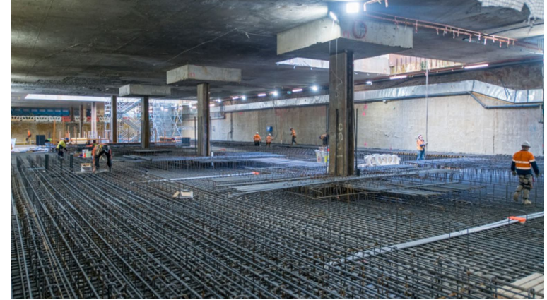
South box concourse slab
