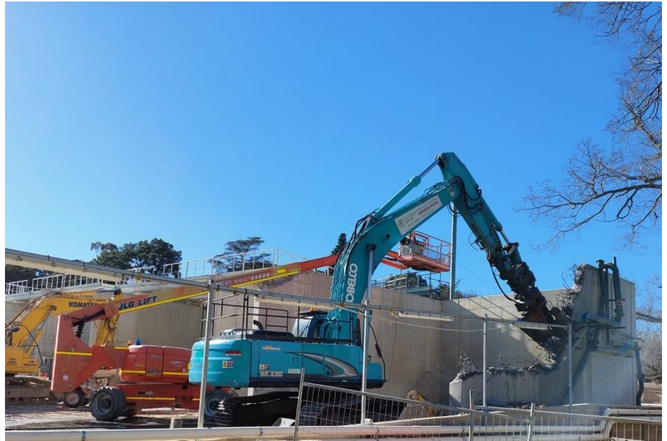
Filter Press bays are demolished
