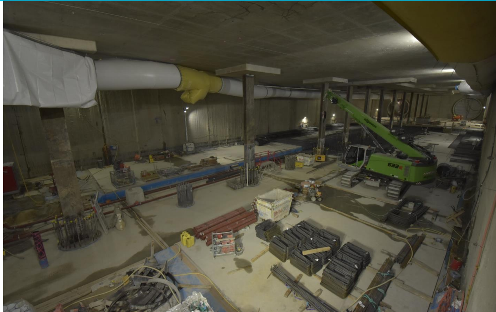
Base slab works underway in the south box
