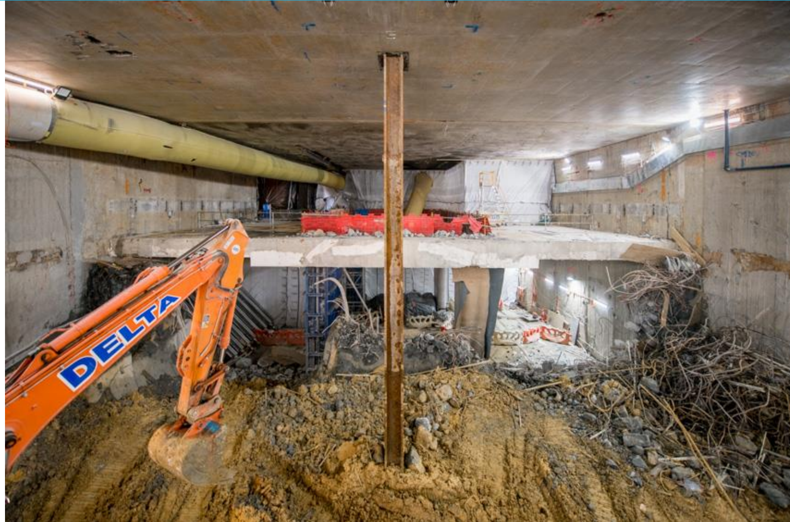
Northern end of the south box – excavation and demolition
