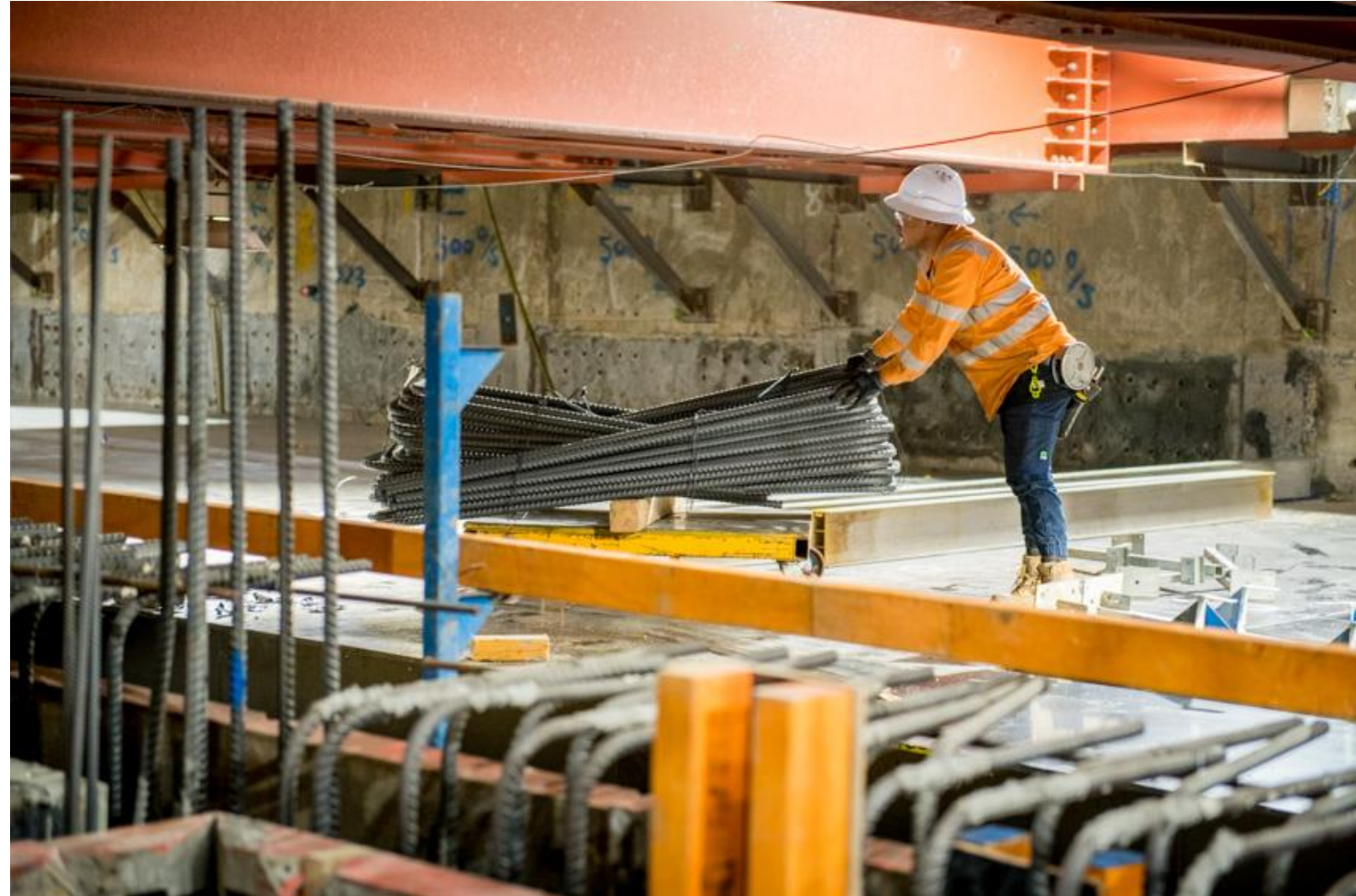
Steel fixing underneath the station support struts
