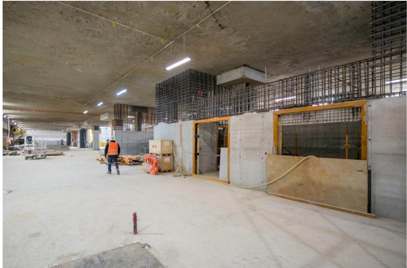
Construction of internal rooms at the concourse level
