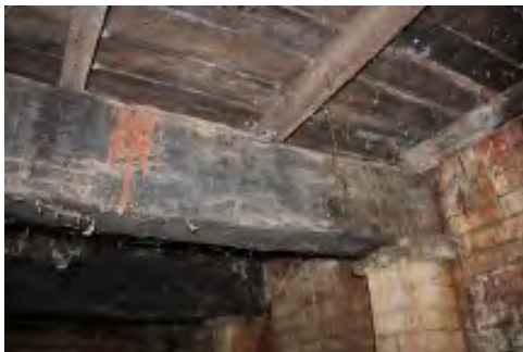
Plate 3: Beams in underground cellar, St Ethel's Winery. Courtesy of Gary Withers, Stawell Historical Society.
