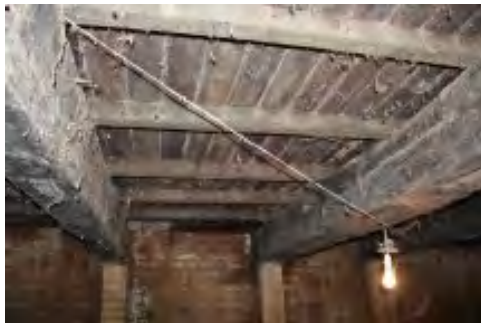
Plate 2: Beams in underground cellar, St Ethel's Winery. Courtesy of Gary Withers, Stawell Historical Society.
