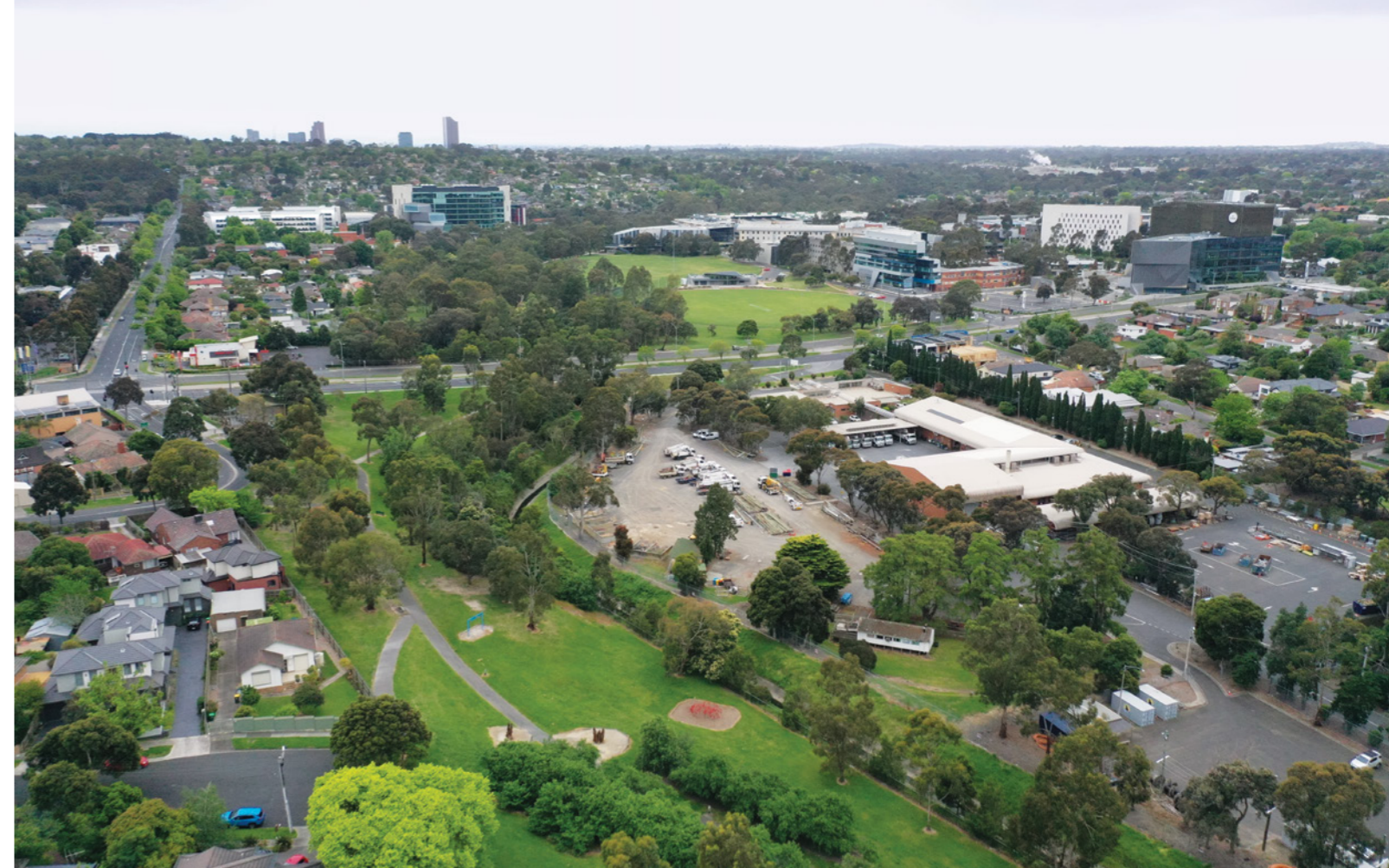
Aerial image of SRL East station precinct at Burwood
