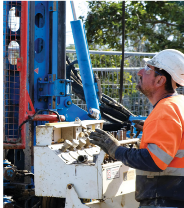
SRL East site investigations at Burwood
