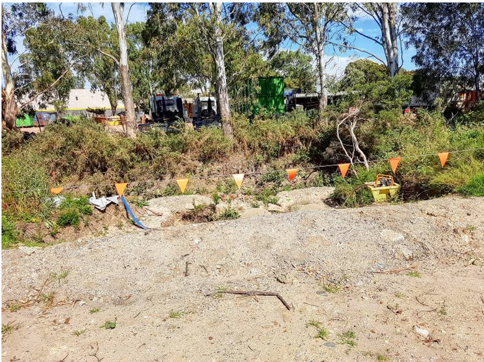
Above: The drainage area further south of Lower Dandenong Road has been bunded, preventing any runoff entering the area directly.
