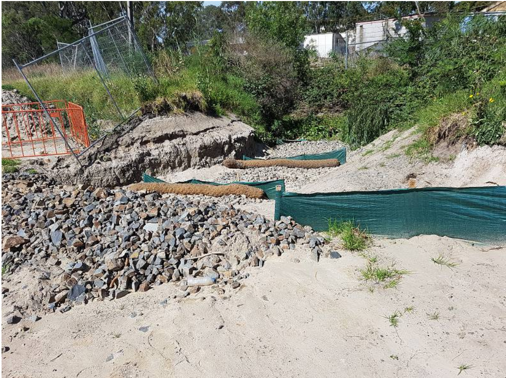
Above: The area immediately south of Lower Dandenong Road. Sediment fences and coir logs have been installed to slow down runoff water. Ballast filled trenches have also been installed to further slow down the runoff and collect sediment.
