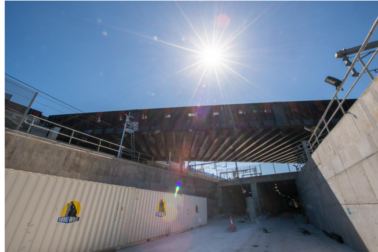
Material will be lowered off the William Street Bridge
