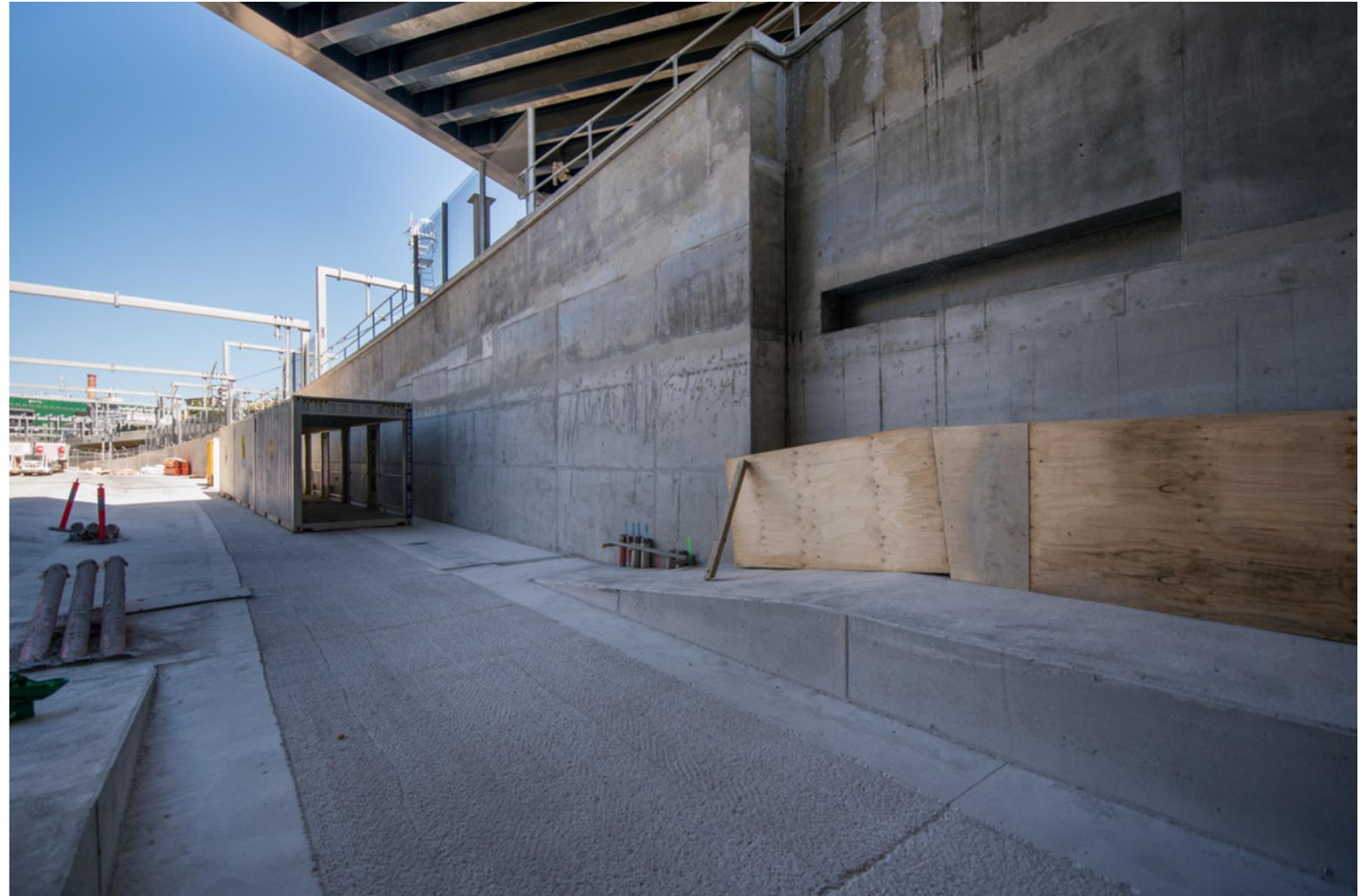
Concrete trackform in decline structure
