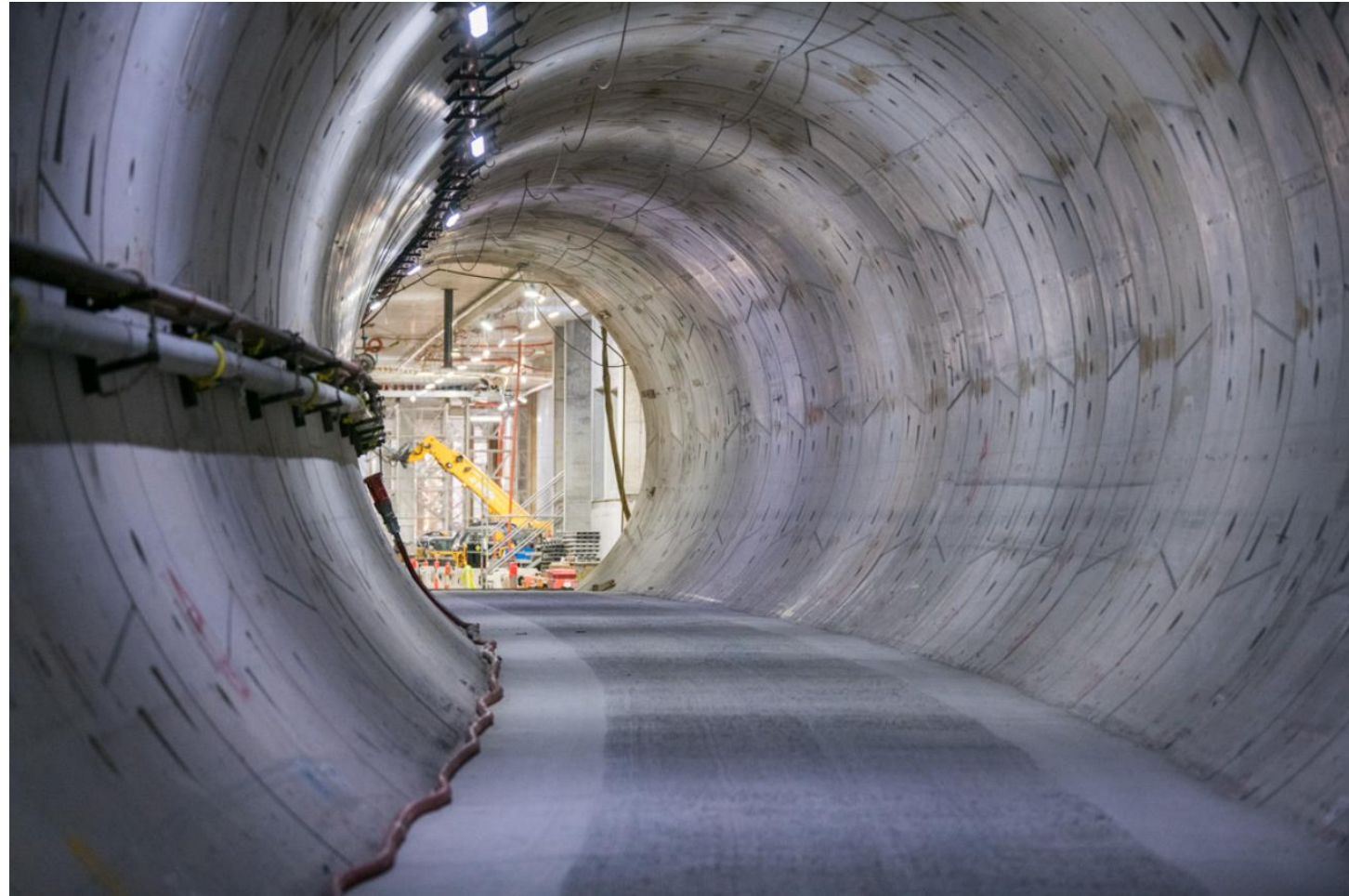
Tunnel Leading to Anzac Station
