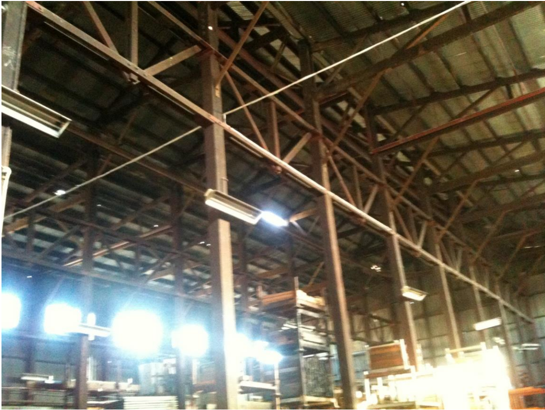
Image 2: Interior of the shed that is unaddressed in the EES.
