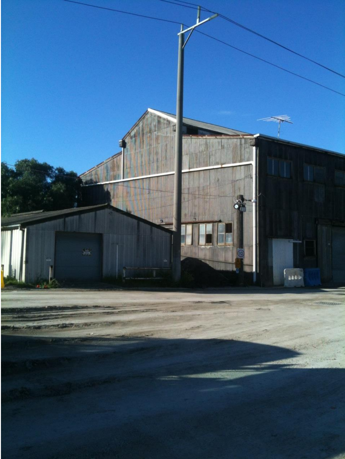
Image 1: The eastern end of the shed to the immediate west of the recommended HO1093.
