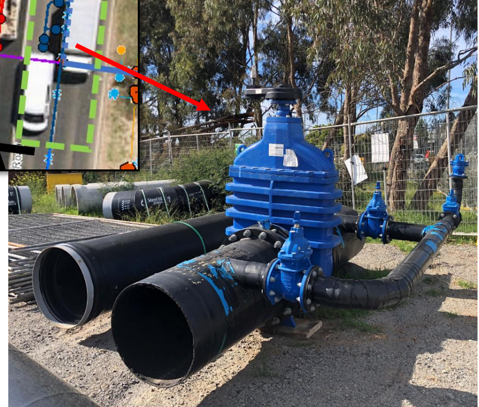
Dn600 Isolation Valve and Bypass Dimensions: 2160mm high, 1700mm Wide Installed 3m deep
