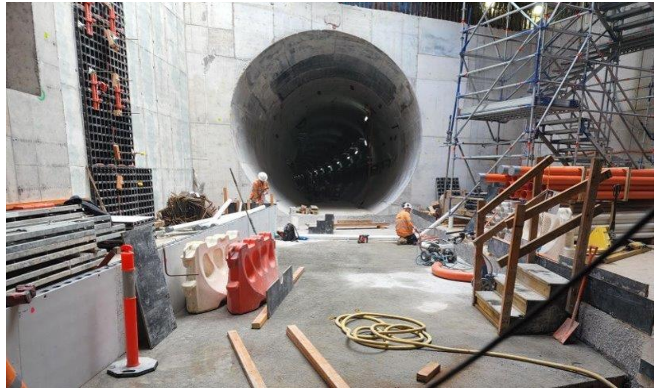
Completed stub tunnel
