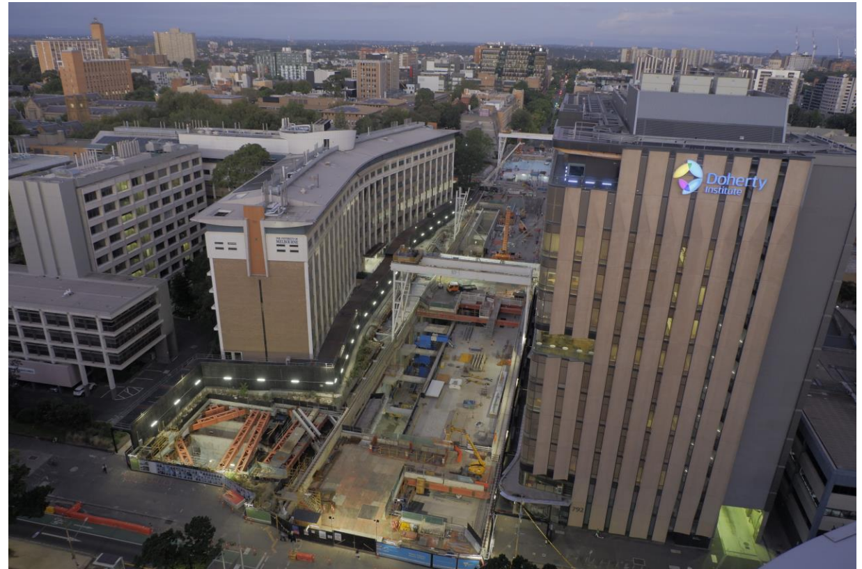
Gantry crane removal
