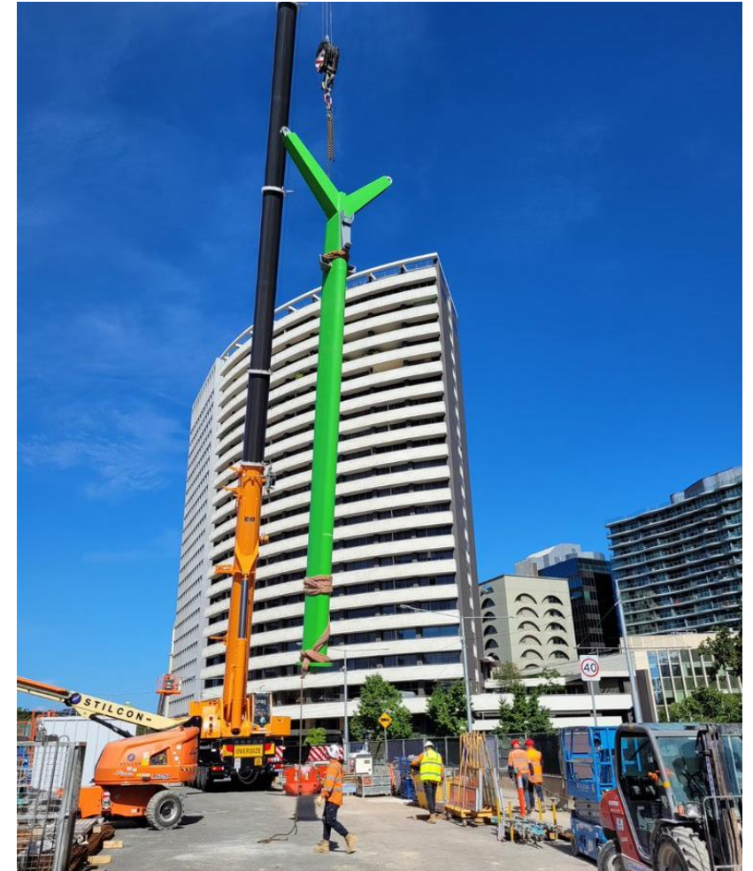
Anzac Station canopy leg being lowered
