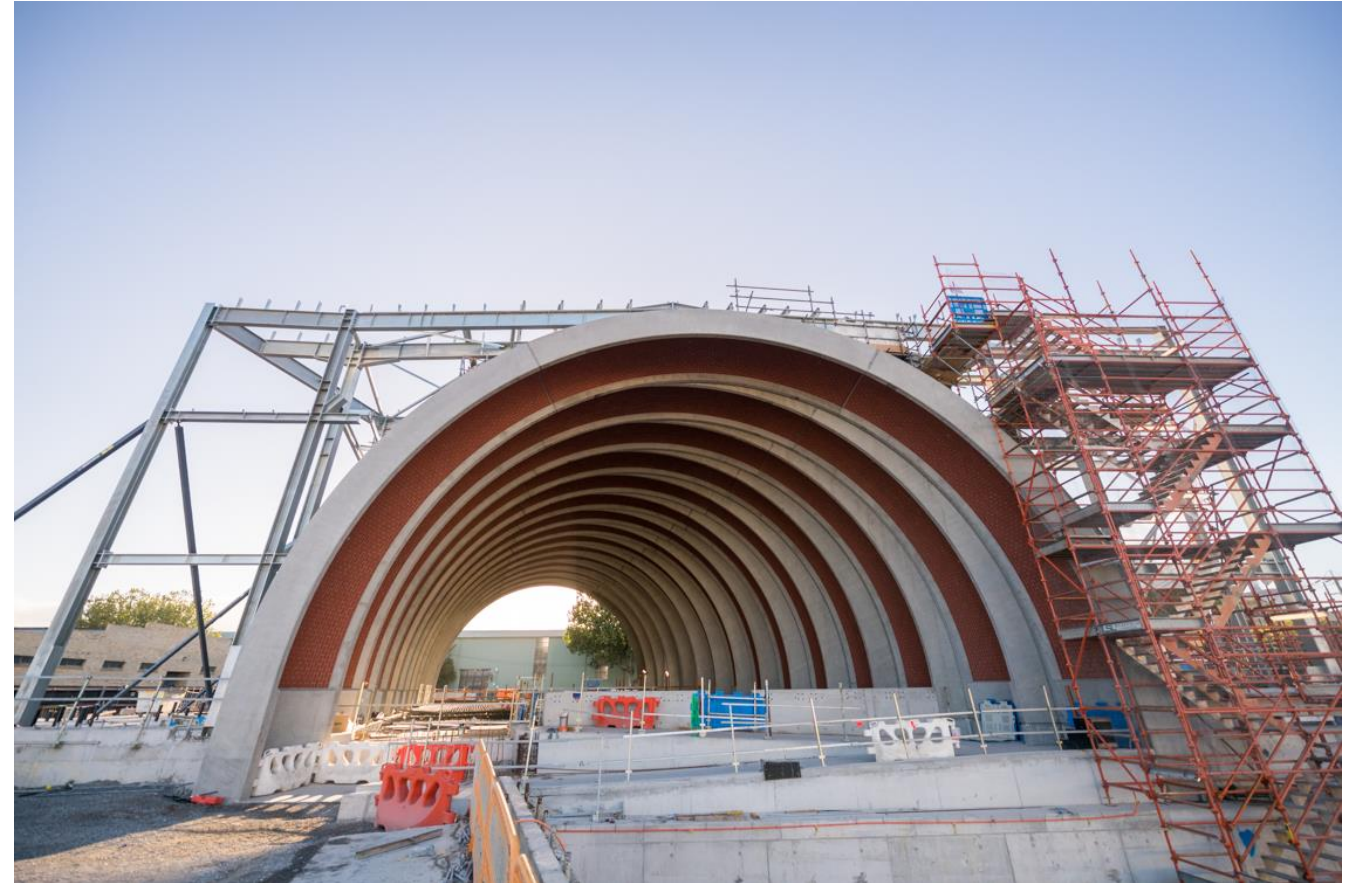
Structural steel installation for station entrance building
