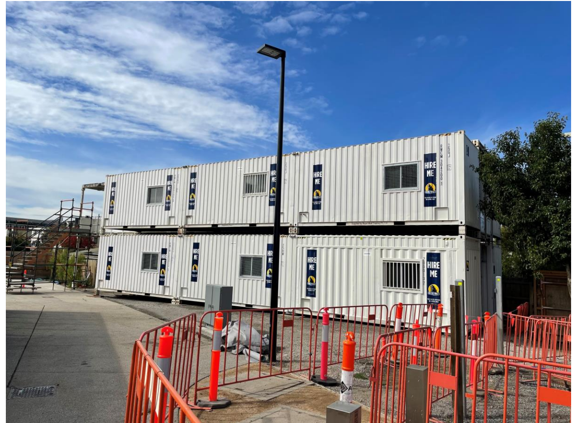
Installation of site facilities on William Street
