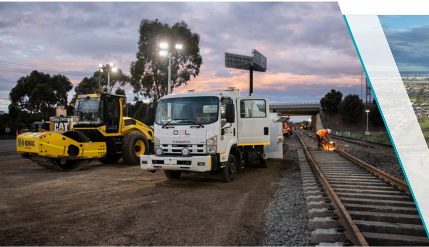
Works get underway in the Fitzgerald Road rail corridor
