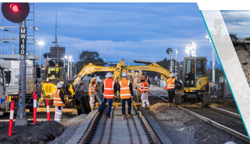
Construction crews survey the rail
