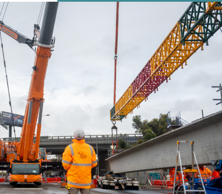
The 750-tonne crane in action
