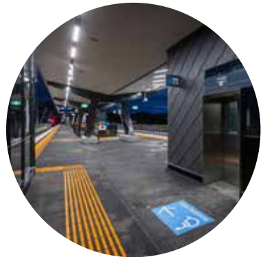
The new platform and station finishes
