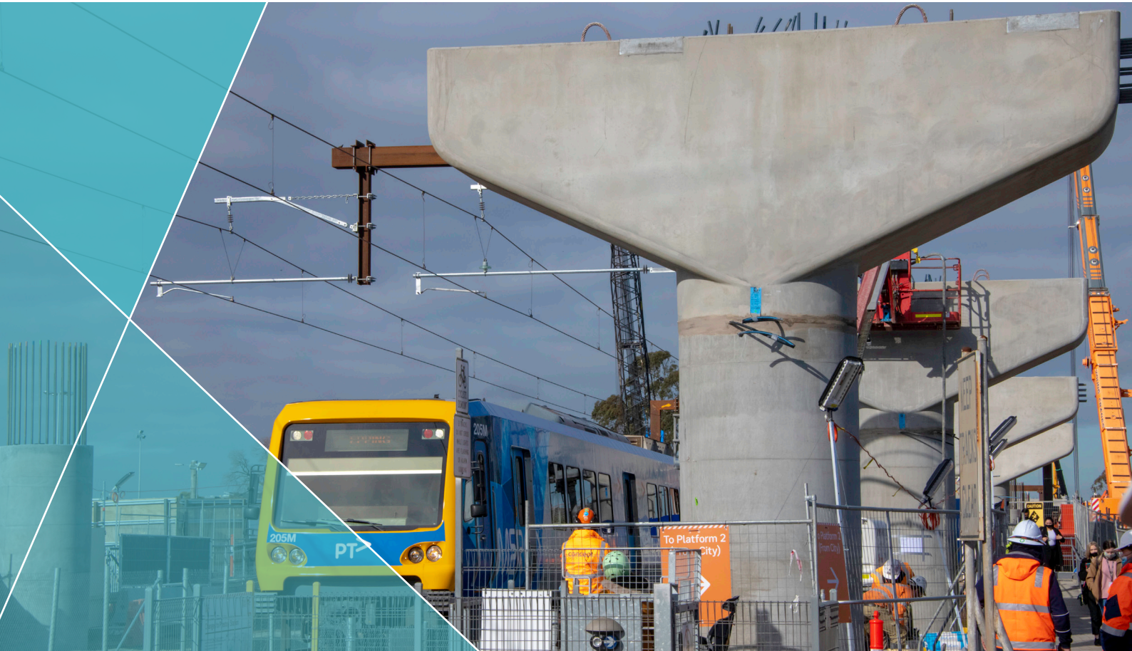
Rail bridge under construction at the Preston Level Crossing Removal Project
