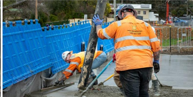
Workers pouring concrete for the new Platform 1 at Montmorency Station
