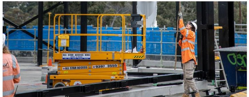
Installation of structural steel at the new Greensborough Station
