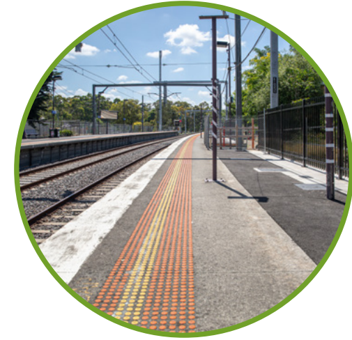
Platform two extension at Diamond Creek Station
