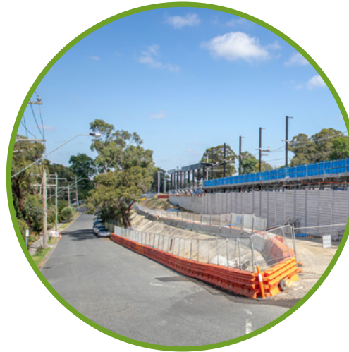
New Montmorency Station view from Station Road
