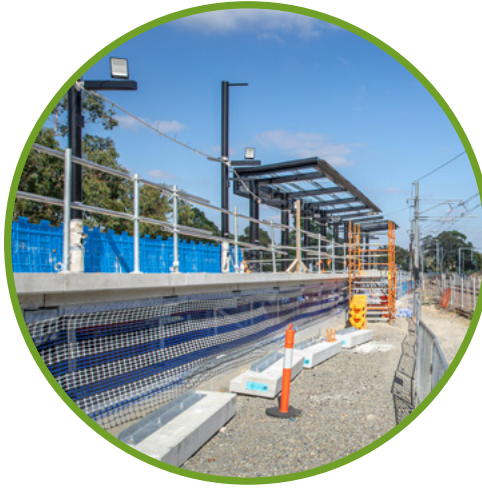
Platform works at the new Montmorency Station
