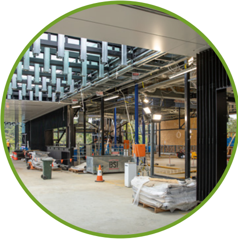
Interior of the new Greensborough Station taking shape
