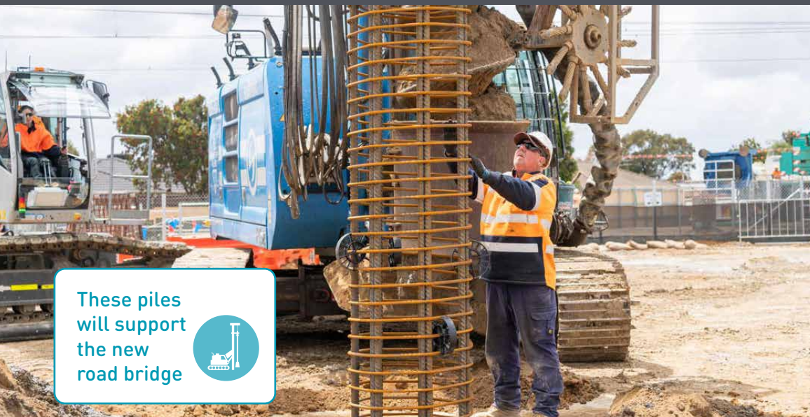
Pile cage being lowered.
