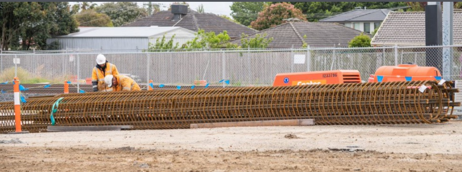
35 pile cages were installed at Camms Road.
