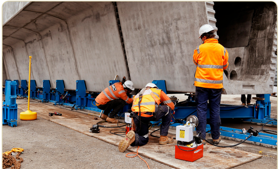
Workers interlocking segments on jacks in the assembly area.
