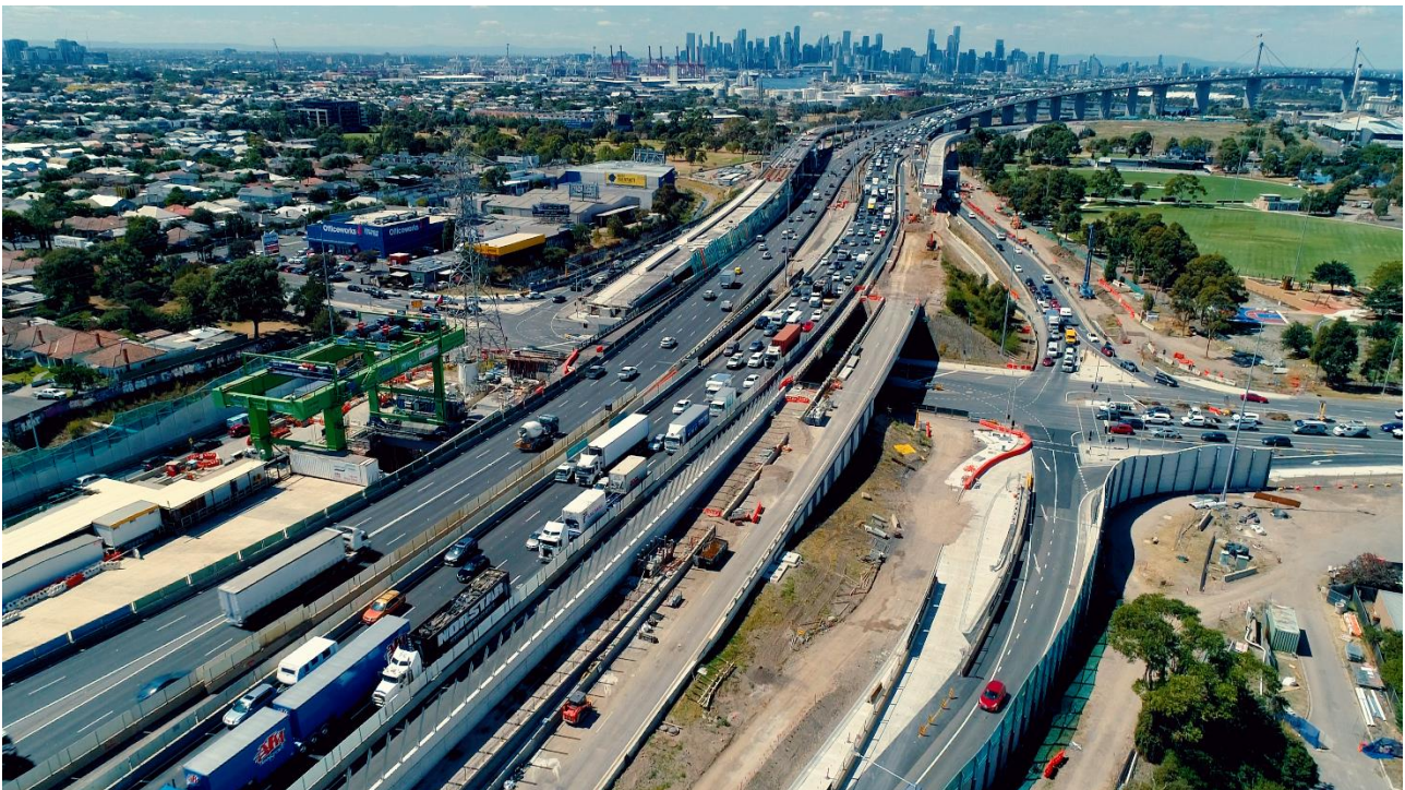
Photo 7 – Williamstown Road Interchange – West Zone (Source: WGTP MTIA, 20 March 2023)
