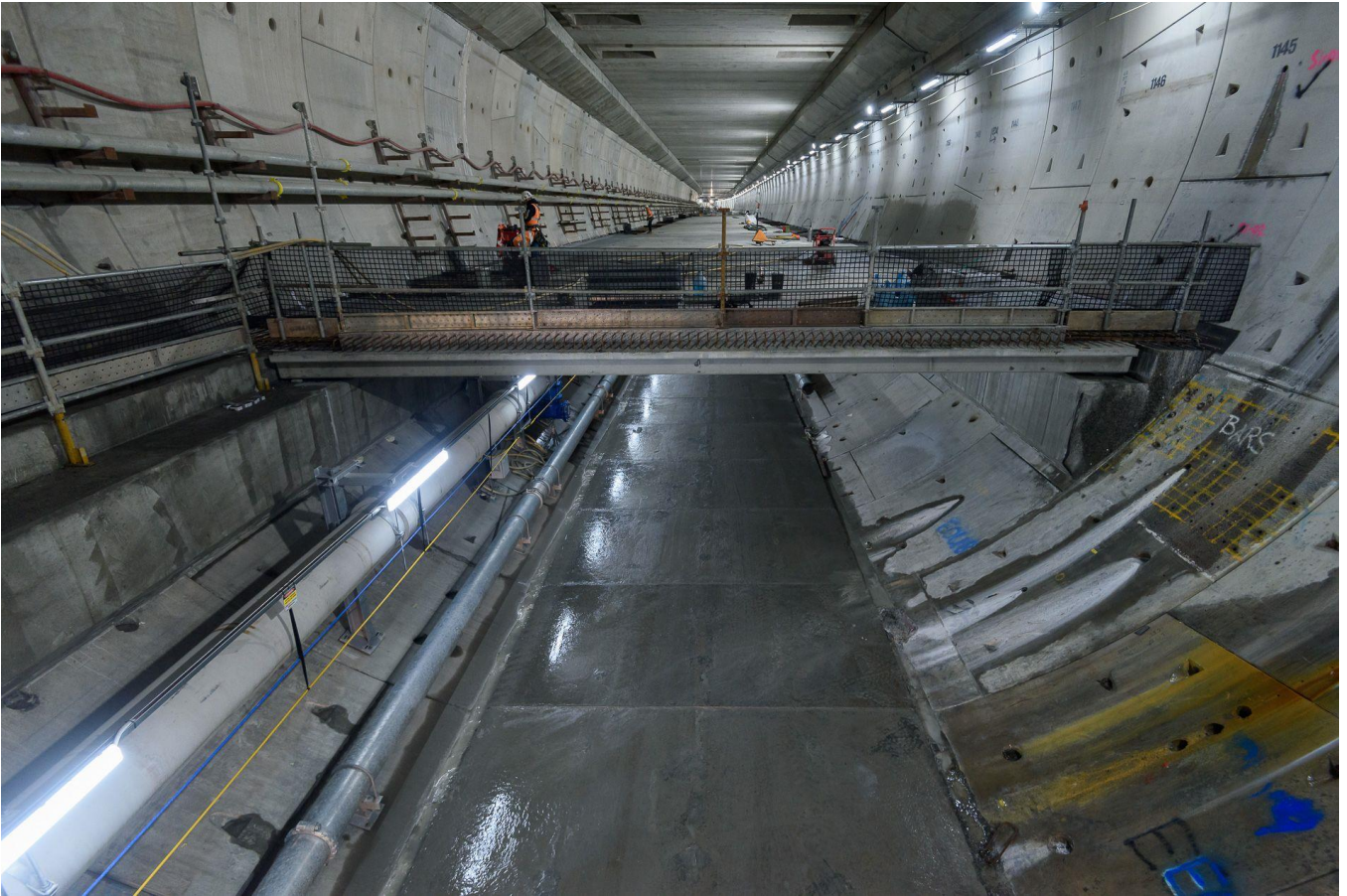
Photo 1 – Tunnel Zone (Source: WGTP MTIA, 8 March 2023)
