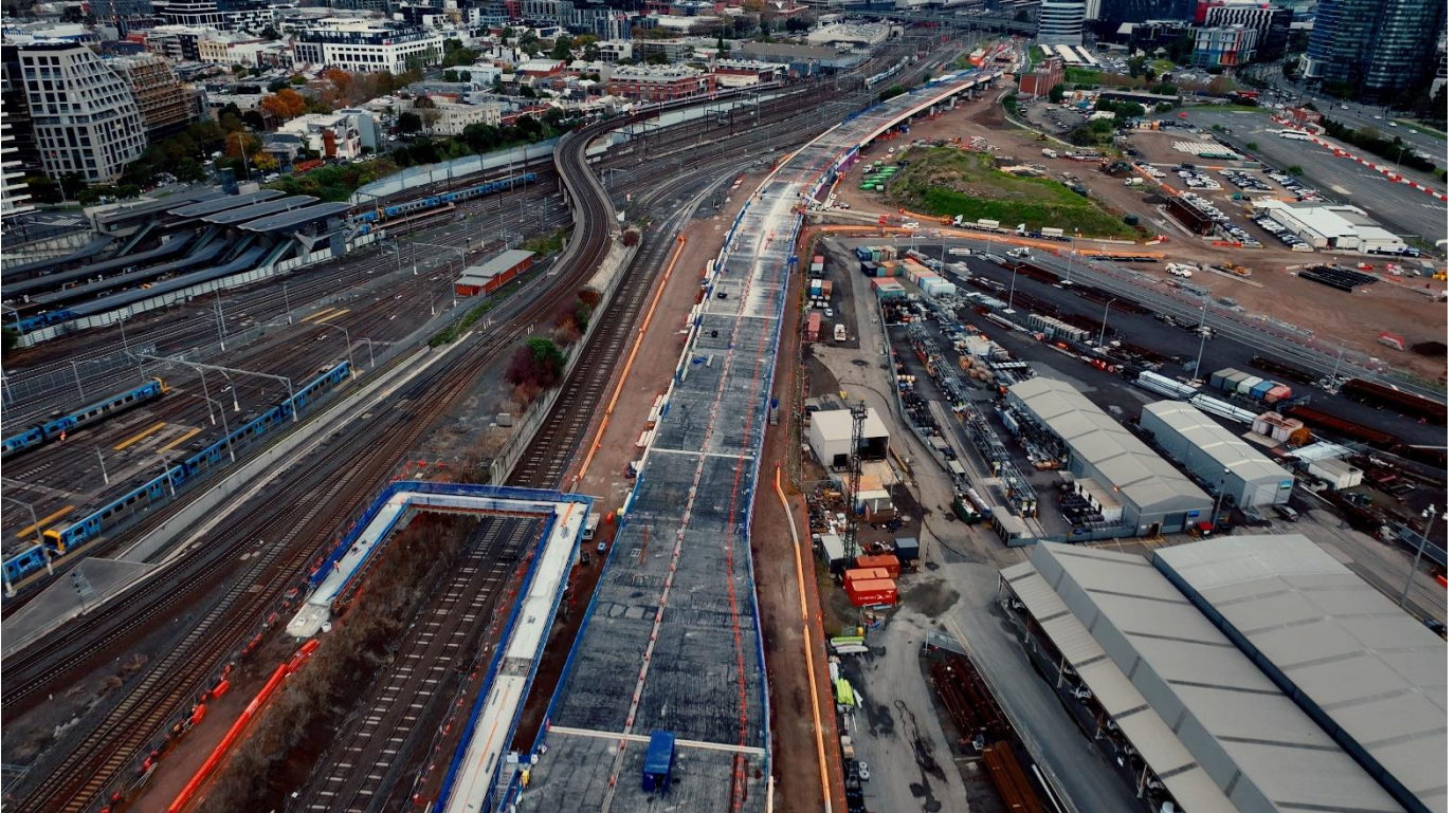
Photo 5 – Wurundjeri Way – East Zone (Source: WGTP MTIA, 6 June 2023)
