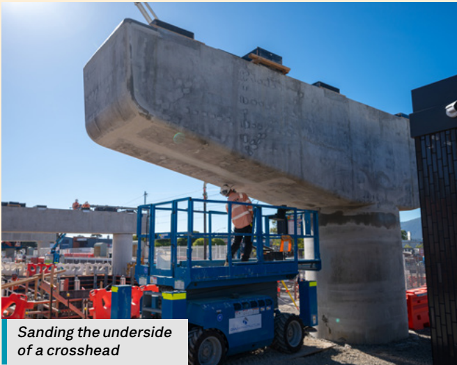
Concrete pumping and crosshead construction in Croydon
