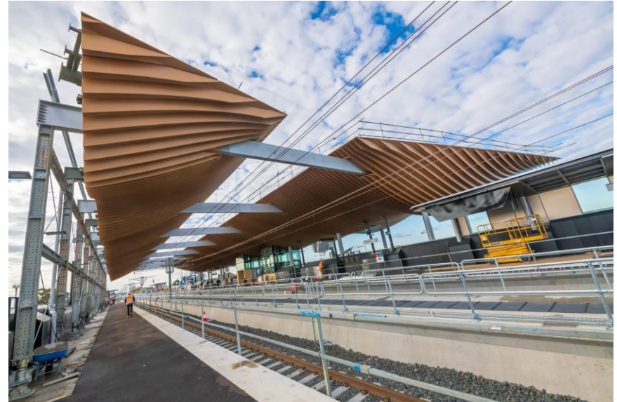
View of station canopy being installed from platform 2
