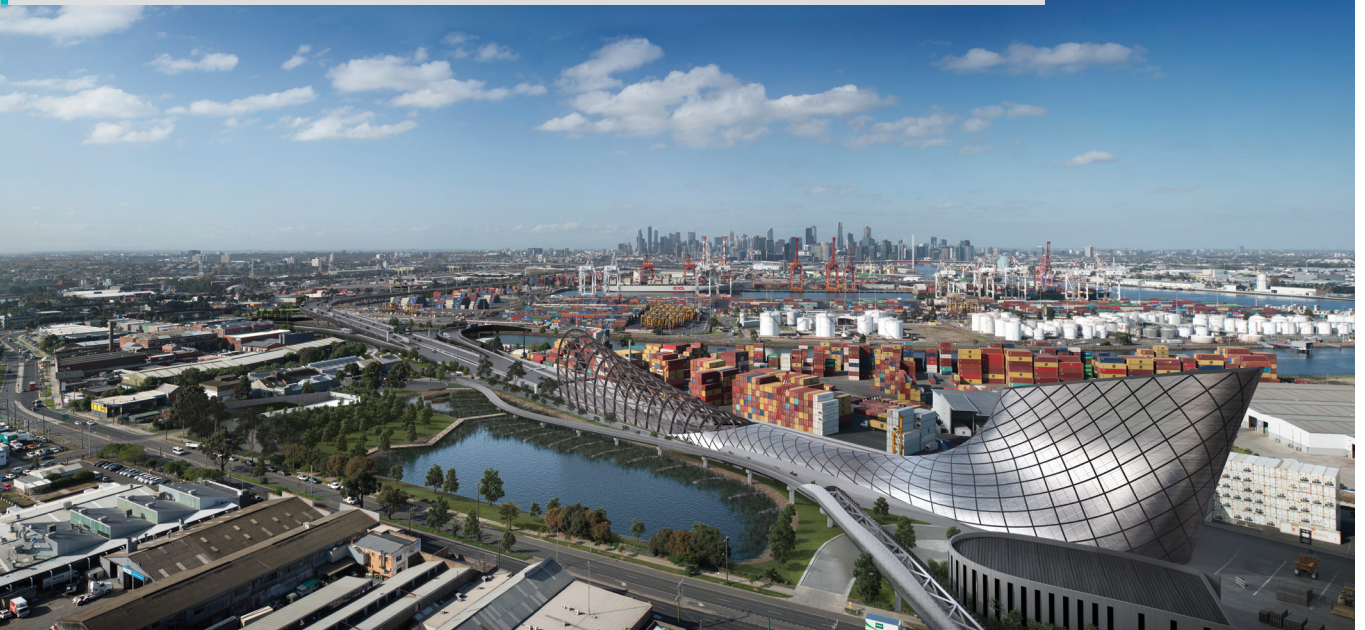
Artist impression of the Yarraville tunnel entry and exit ventilation structure and timber net structure
