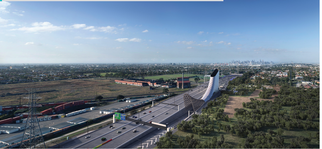
Artist impression of the outbound tunnel exit ventilation structure and timber net structure
