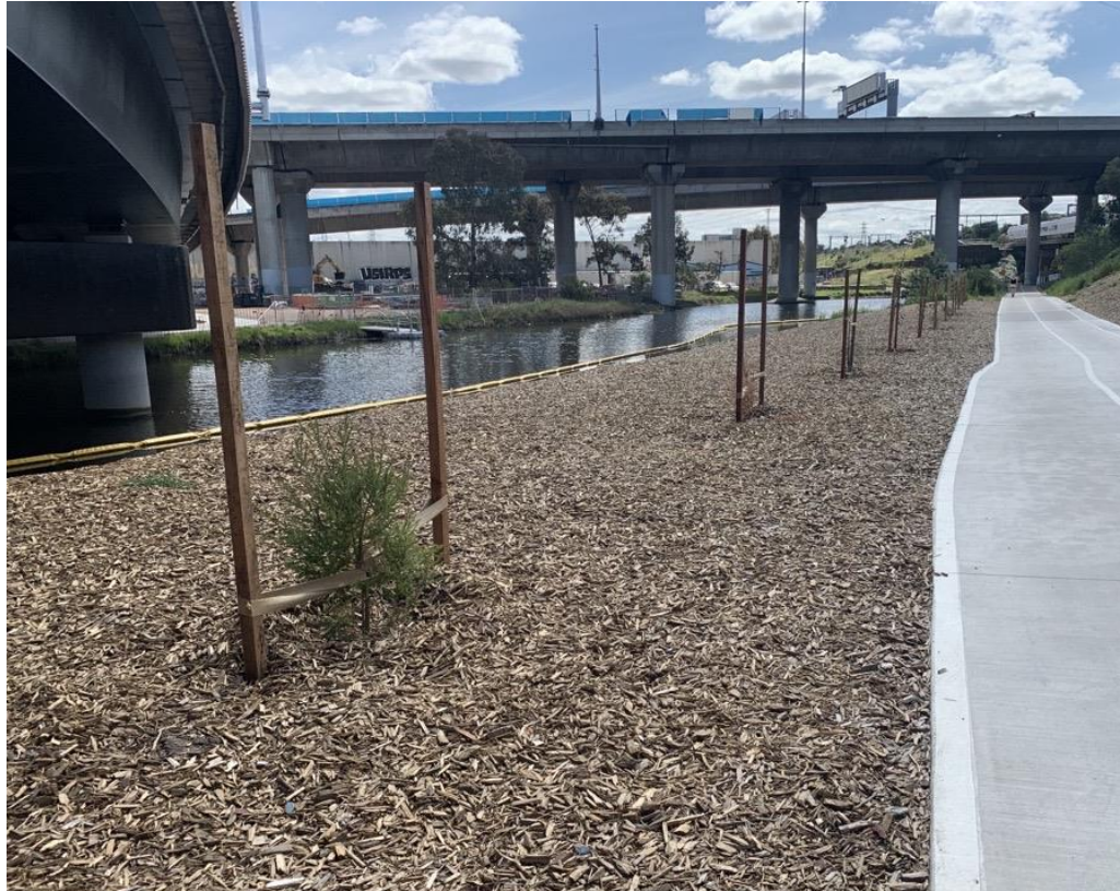
Landscaping along the Moonee Ponds Creek Trail
