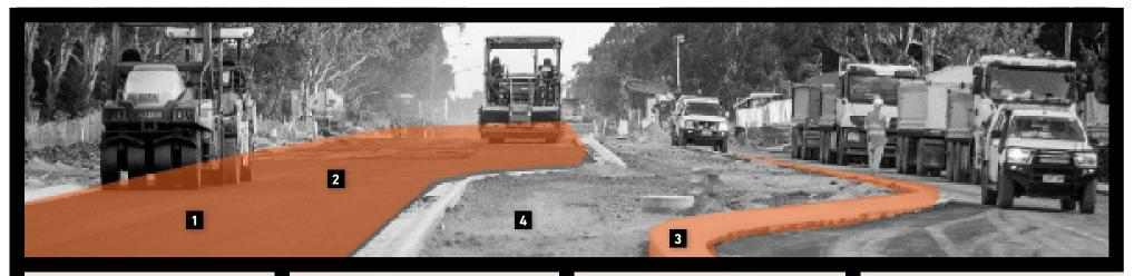
Warm mix asphalt is heated to lower temperatures (~150°C vs 175°C) resulting in reduced emissions (~4%). Together with high RAP content results in lower carbon pavements. Consider also, 'ultra low' warm mix asphalts which are produced at even lower temperatures (~110°C) and could potentially be heated using fossil fuel free energy sources.
