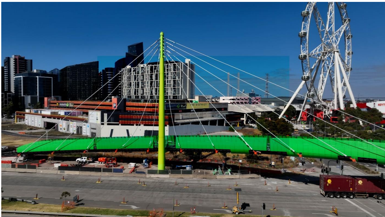
Photo 4 – Footscray Road – East Zone (Source: WGTP MRPV, 4 March 2024)
