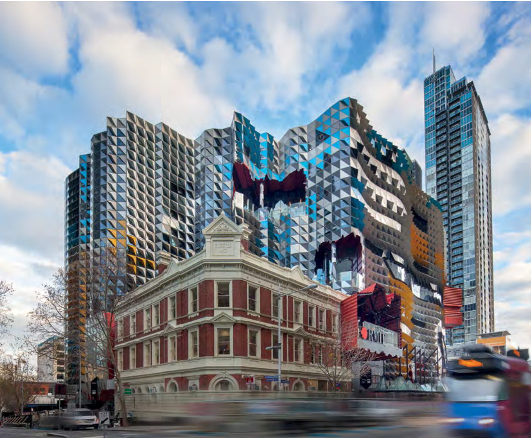
The Oxford Scholar Hotel and RMIT University's Swanston Academic Building, at the corner of A'Beckett Street and Swanston Street, Melbourne (see 4.5.3). The relationship between new development and historic corner pub is very similar to the over-site development opportunity in the Cocker Alley sub-precinct at the CBD South station (see 4.6.1).
