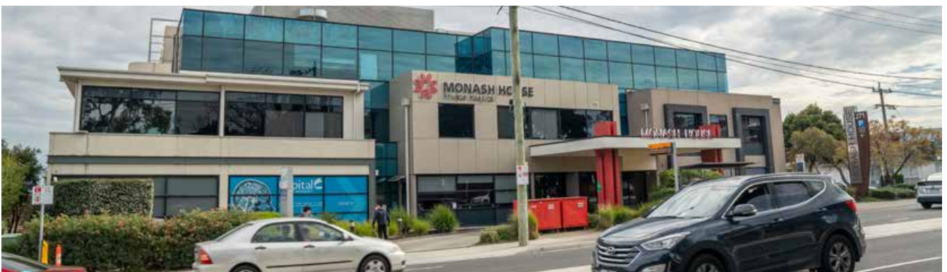
Monash House Private Hospital
