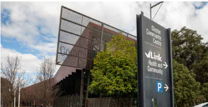
Clayton Community Centre
