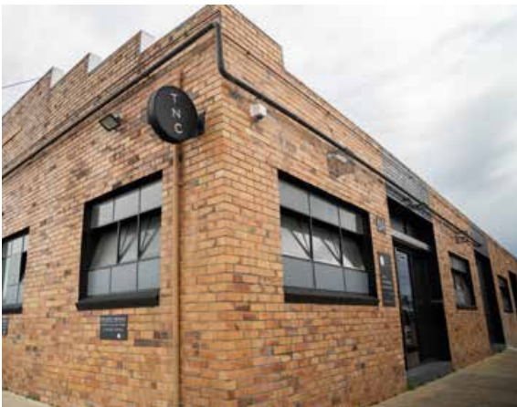
Upgraded warehouse, Clayton
