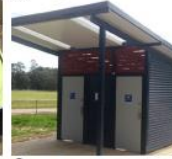
4 New Toilet Facilities
