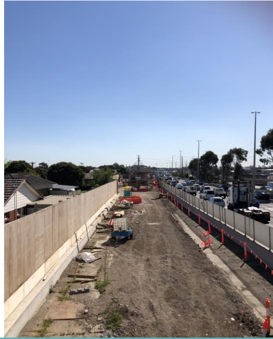
Outbound widening works – looking west
