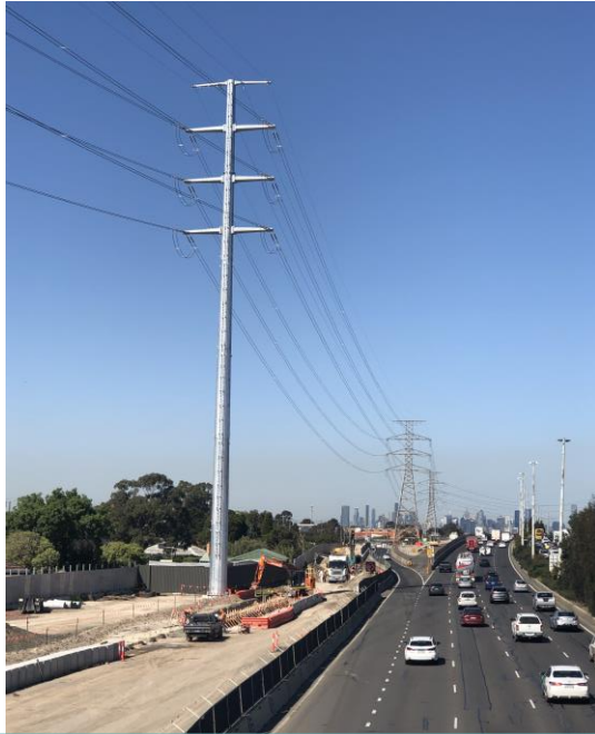
Inbound widening works – looking east
