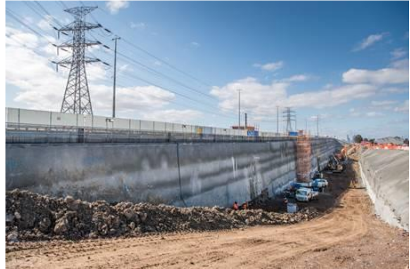
Outbound southern portal works
