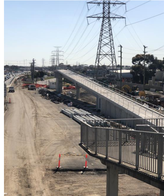
Rosala Avenue ramp for new walking and cycling overpass
