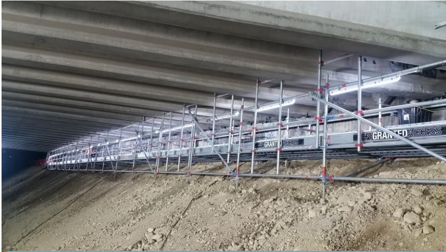
Beneath Kororoit Creek bridge – lifting bridge up to strengthen and widen
