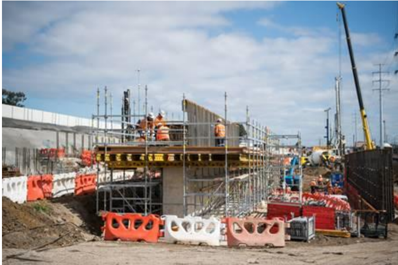
Inbound southern portal works
