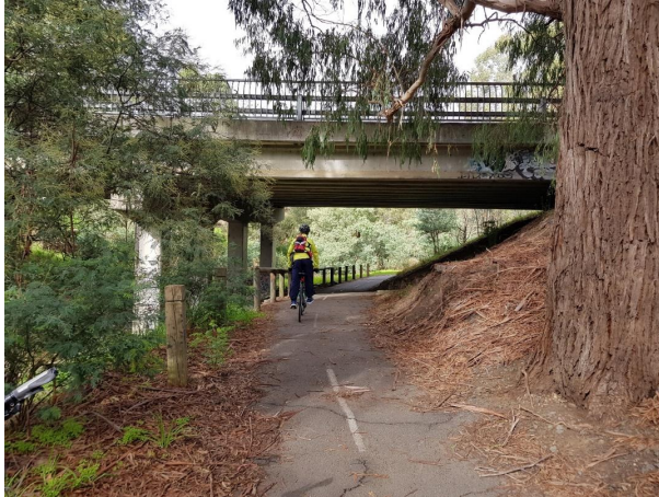
Figure 94 Plenty River Trail at Main Road
