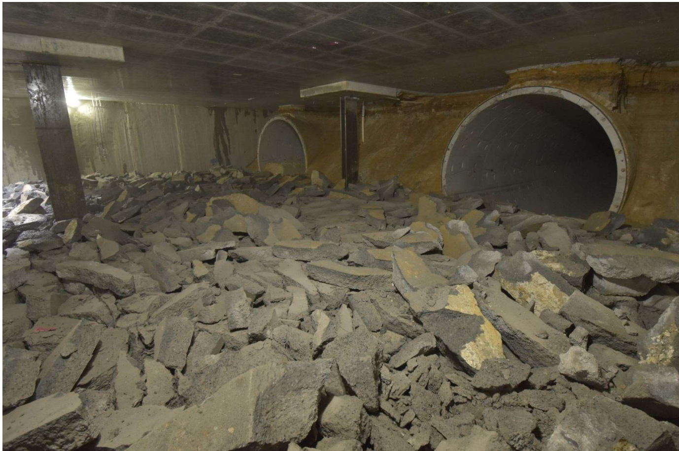
Stage 2 excavation underway on the sacrificial tunnel (27 April)
