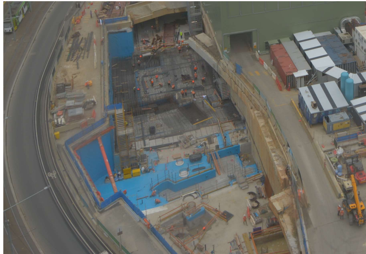
Steel fixing moving from north to south in the tram box
