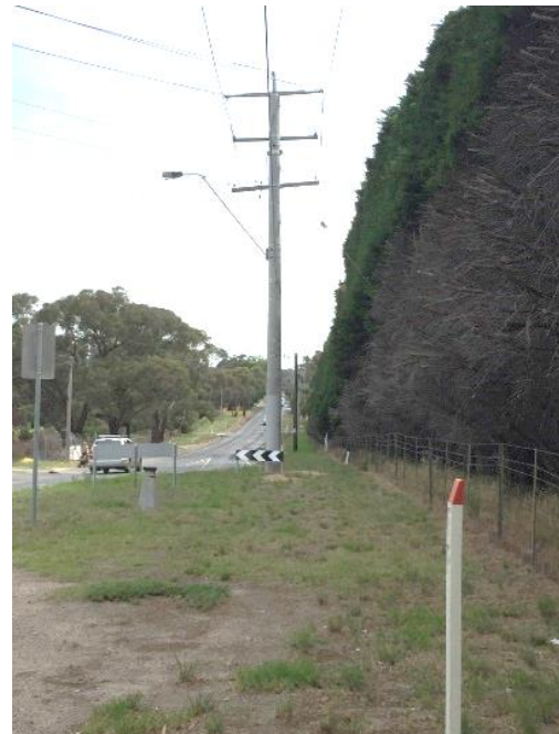
Plate 58: Disturbance from installation of underground services, facing north (Minos 18.12.2017)
