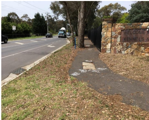
Plate 18: Project area at corner of Yan Yean Road and Ashley Road, Yarrambat, facing south, showing the pedestrian path and underground services (Minos 2017)
