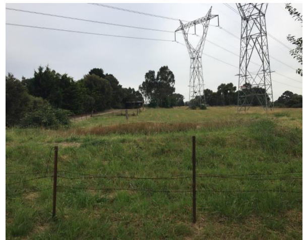
Plate 75: Easement for installation of services, facing north from Bridge Inn Road (Minos 18.12.2017)
