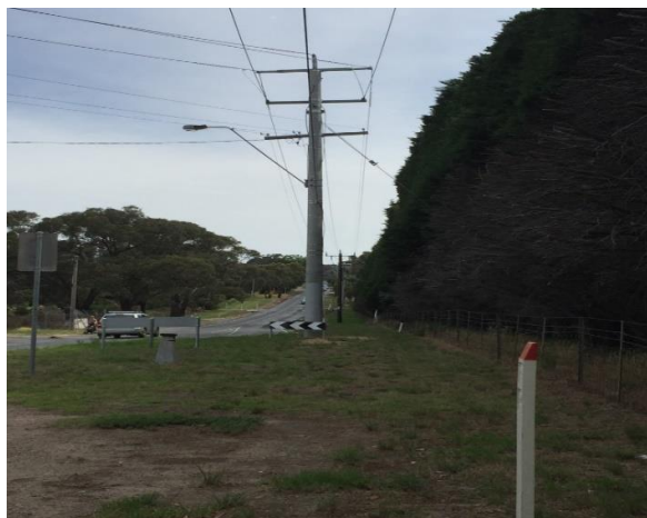
Plate 12: Project Area, facing north showing overgrown mature conifers (Minos 2017).
