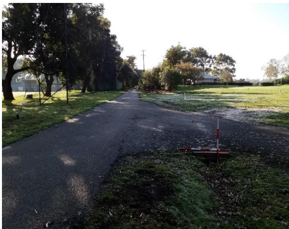
Plate 29: Sealed pathway present across entirety of Yarrambat Golf Course, facing west (Russell 2020)
