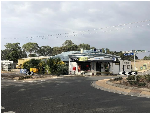
Plate 3: Former Post Office and General Store on the south-east corner of Yan Yean and Doctors Gully Road, facing southwest
