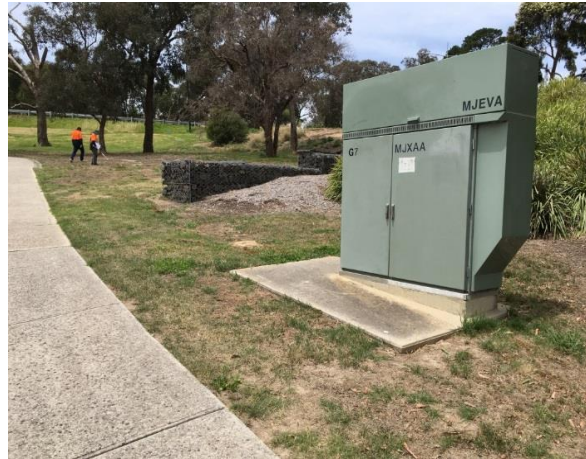
Plate 36: Project area north of Jorgensen Avenue, showing evidence of subsurface services and landscaping, looking east towards Yan Yean Road embankment (Minos 2017)
