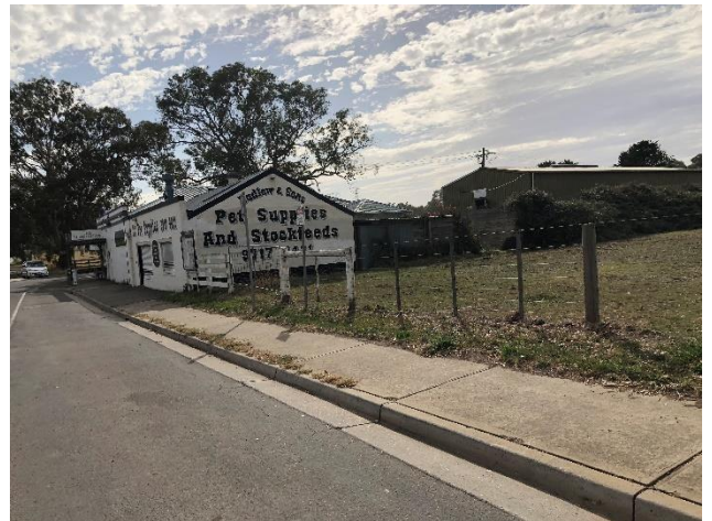
Plate 4: Rear of the Former Post Office and General Store, facing east.
