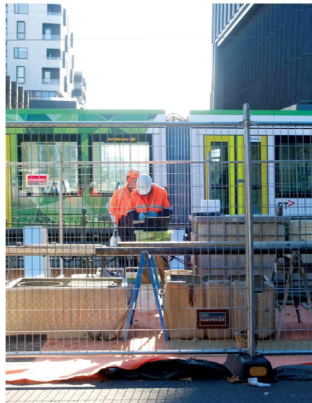
SRL East site investigations at Box Hill
