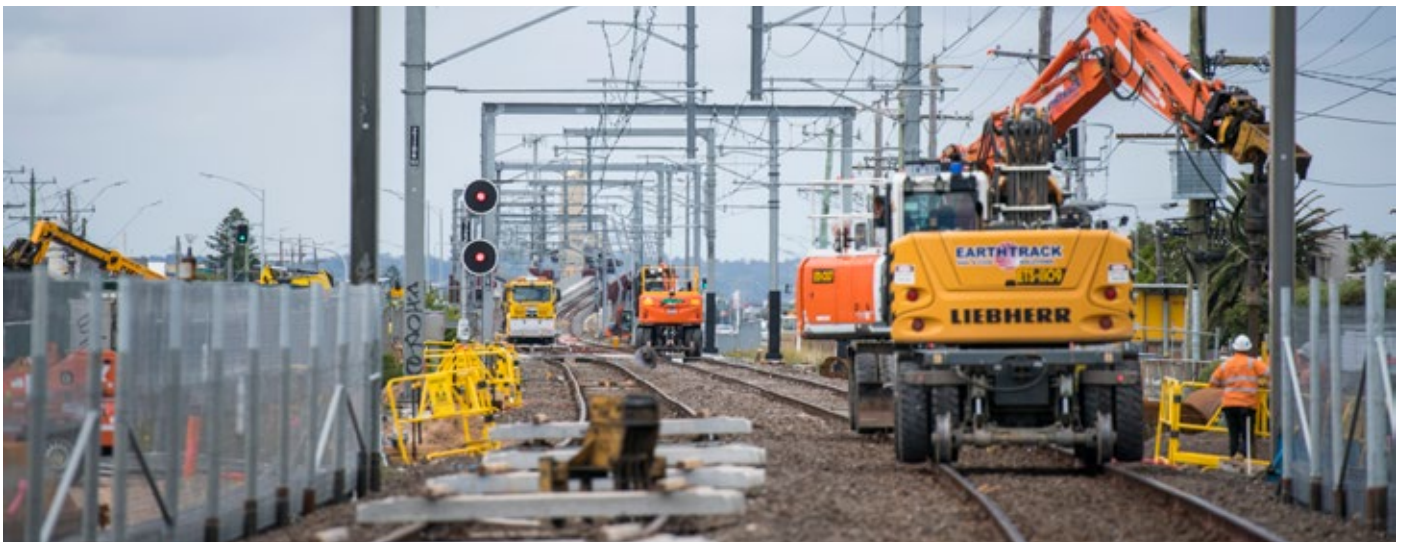
Crews replacing rail sleepers along the rail line between Edithvale and Bonbeach during our February rail closure
