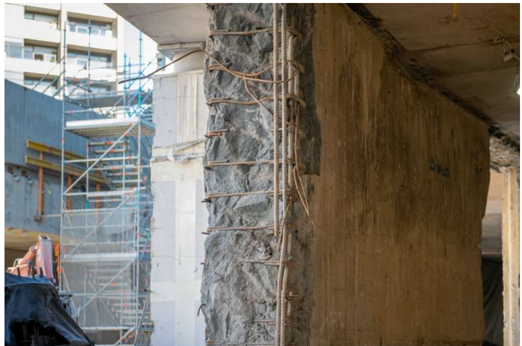
D-wall demolition – tram interchange to concourse
