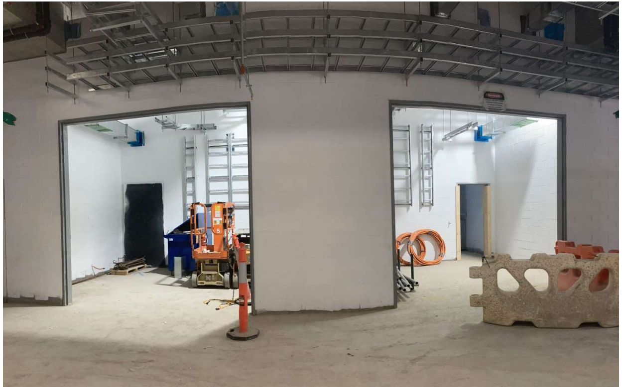
Internal rooms taking shape
