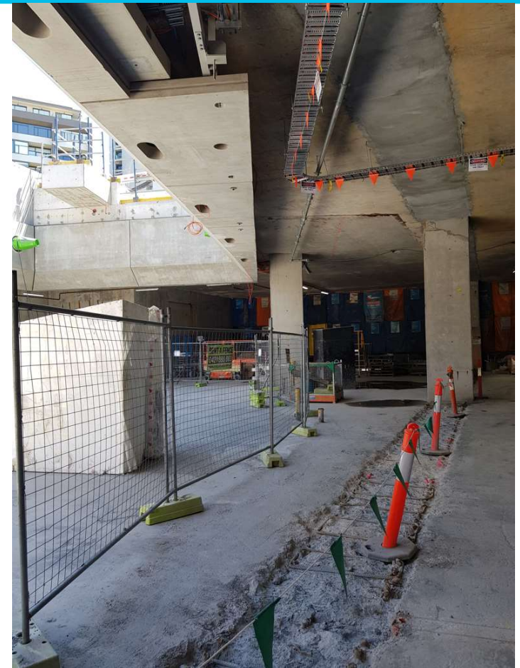
Demolished D-walls and L-shaped precast panel installation
