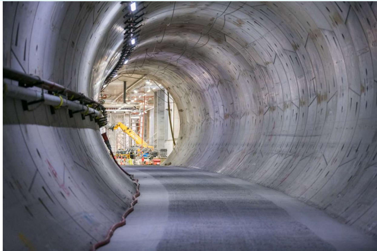
Completed invert concrete leading to Anzac Station
