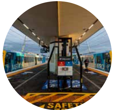
The new platform and station finishes
