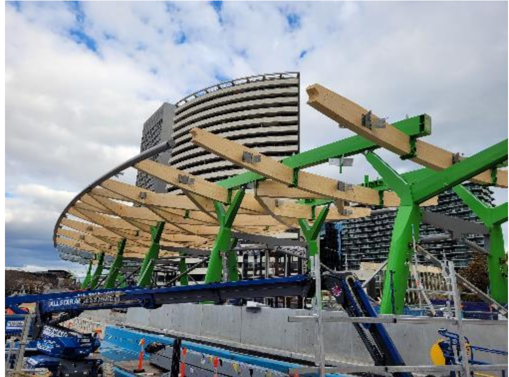
Tram interchange canopy progress
