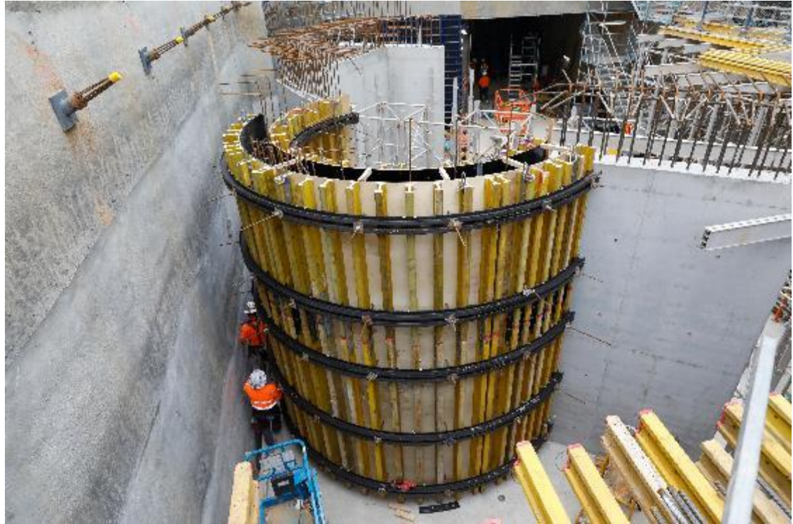
Shrine Entrance - Stage 1 Construction (February 2021)
