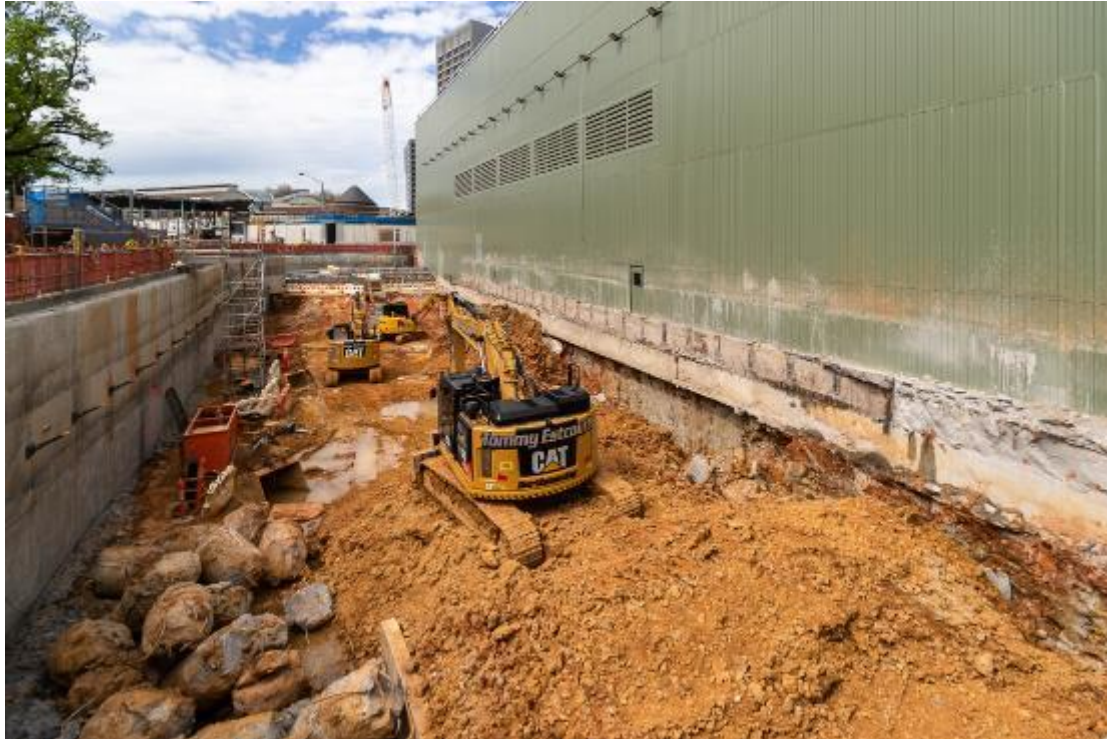
Shrine Entrance - Stage 1 Construction (October 2020)
