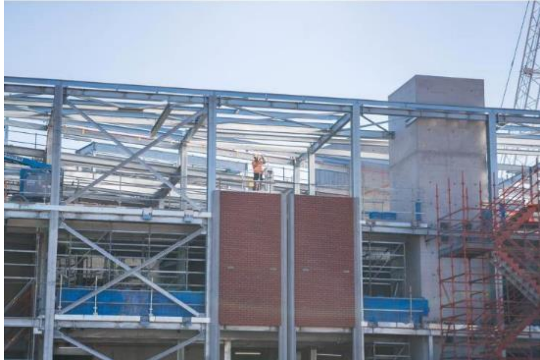
Pre-cast panel installation at Arden Station
