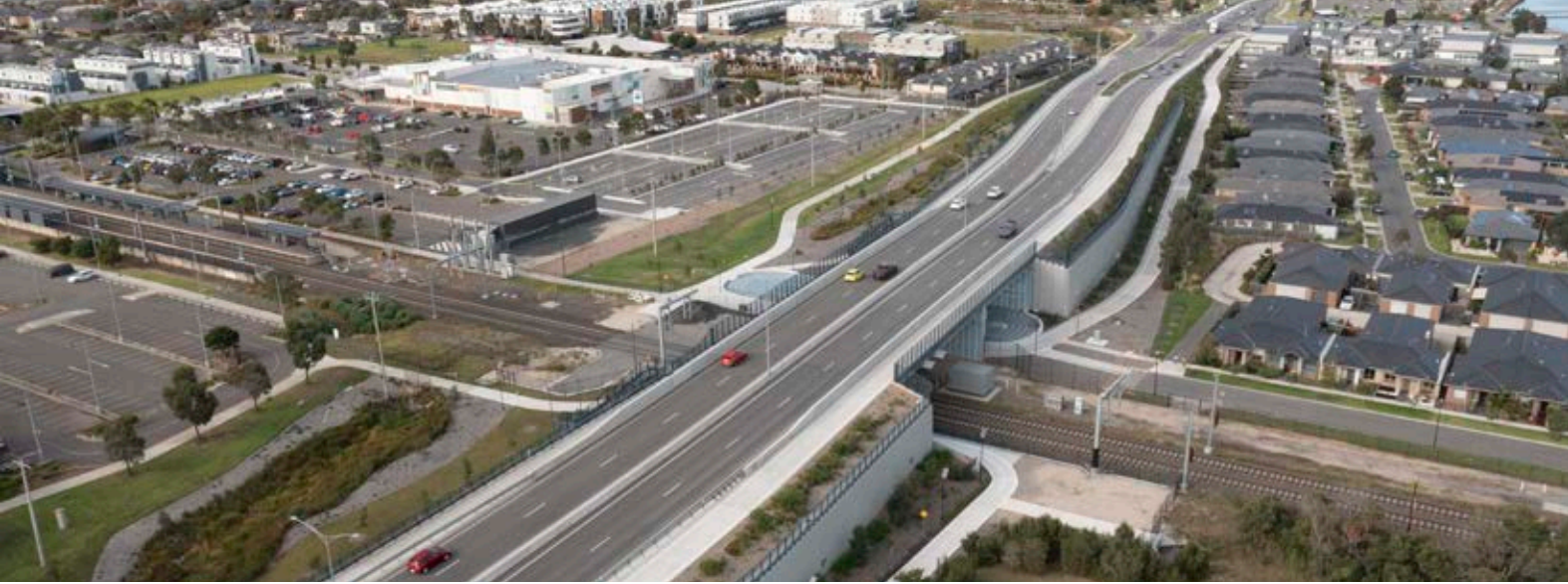
A road bridge over the rail line at Cardinia Road, Pakenham
