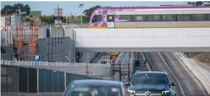
New rail bridge at Robinsons Road
