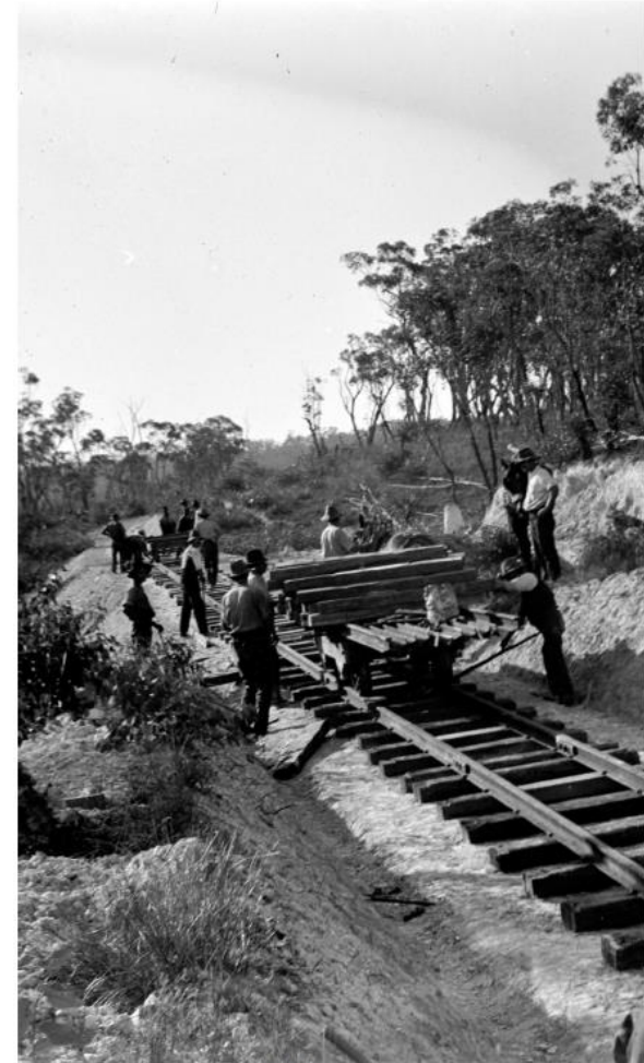
Henty, Wiff, photographer (1901-1940), Railway construction workers laying track through cutting in bush
