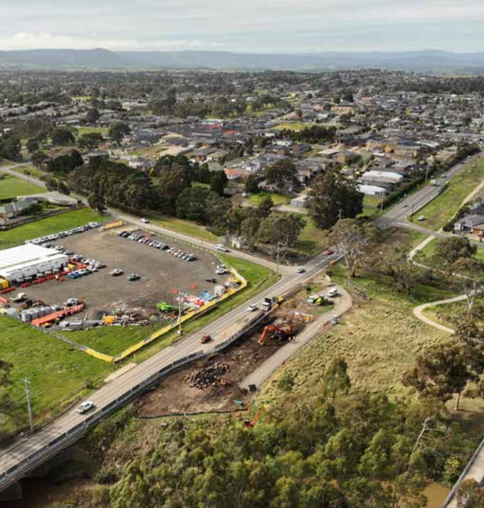
Works are underway to build the new bridge over Plenty River.
