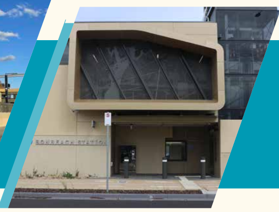
Bonbeach pedestrian overpass screen
