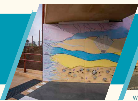
Eel Race Road underpass mural
